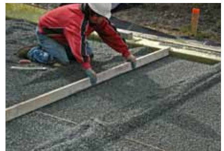
9. Loose screed the clear crushed open-graded bedding course.
