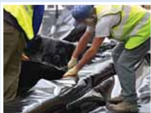
1. Install welded membrane
