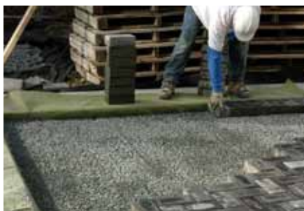
10. Place the AquaPave® pavers.
