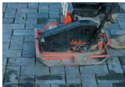
11. Compact the AquaPave® pavers.
