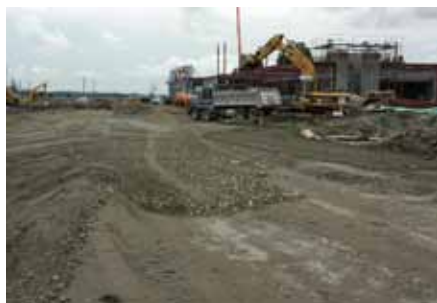
1. Excavate subgrade, removing any organic material.
