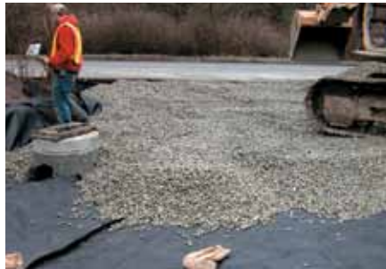
2. Place and spread the clear crushed open-graded lower sub-base aggregate without wrinkling or folding the geotextile.
