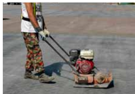
12. After final compaction the paved area is available for immediate use.
