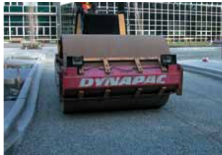
5. Compact the clear crushed open-graded upper sub-base.
