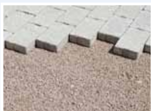
7. Install the AquaPave® pavers
