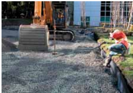
4. Place and spread the clear crushed open-graded upper sub-base.
