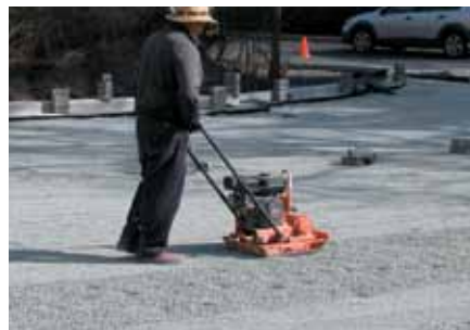
8. Compact the clear crushed open-graded bedding material.
