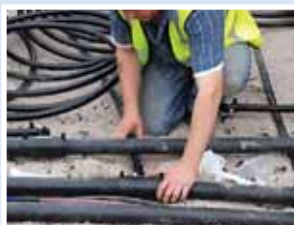
3. Install the geothermal horizontal collector pipes
