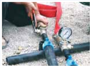
4. Pressurize and system check
