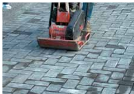
14. Final compaction of the AquaPave® pavers.
