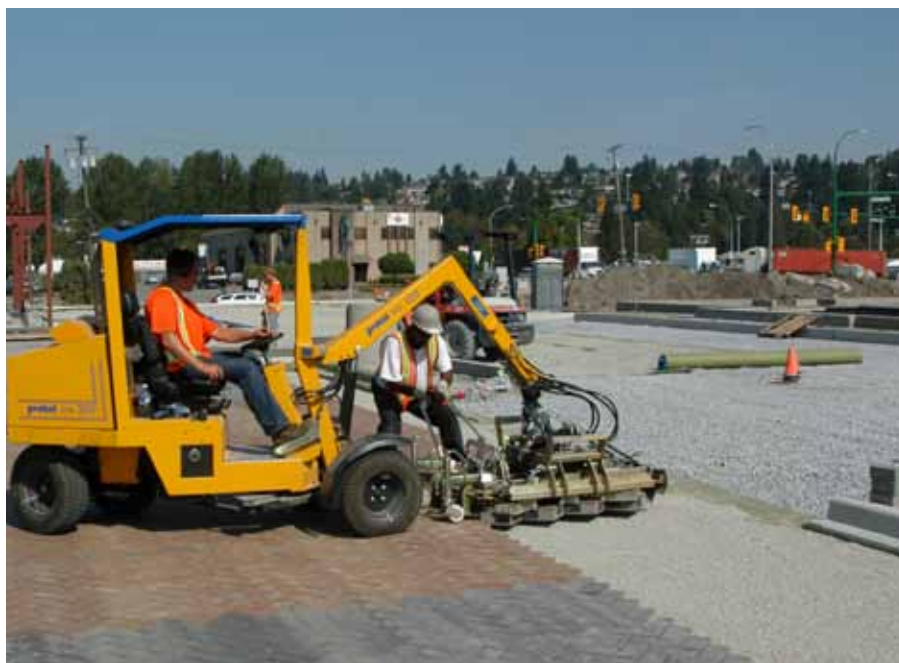
9. AquaPave® is placed using mechanical laying equipment [can increase production to 745-930 m 2 (8,000-10,000 ft 2 ) per day with a standard crew].
