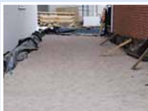
2. Lay and compact 2-6 mm (0-1/4") clean bedding stone
