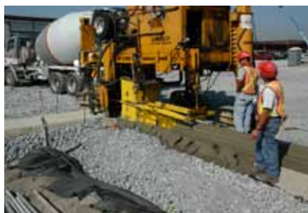
4. Paver restraints are placed.
