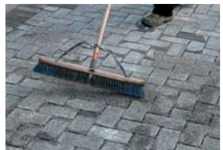
12. Spread and sweep in the AquaPave® Engineered Joint Stabilizer.
