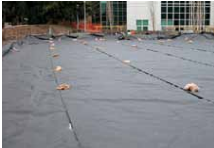
1. Place the AP SC1000 woven geotextile with the specified overlap.
