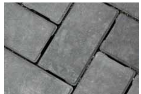
15. Close-up view of the joints with AP Engineered Joint Stabilizer applied after final compaction.
