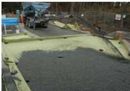
7. Place and spread the clear crushed open-graded bedding material.
