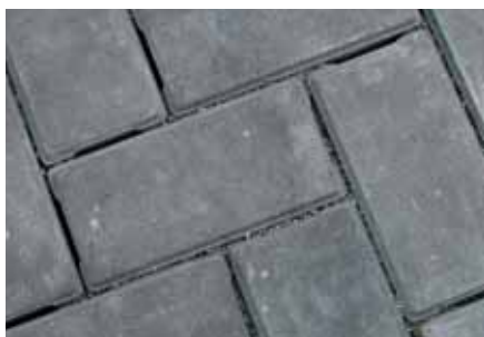
13. Close-up view of the joints with AP Engineered Joint Stabilizer applied before final compaction.
