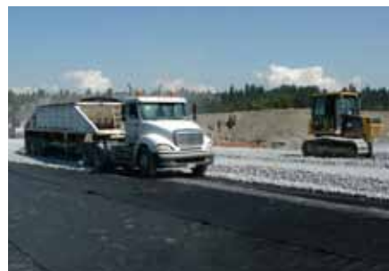
3. Clear crushed open-graded aggregate lower sub-base is placed, followed by grading and compaction.
