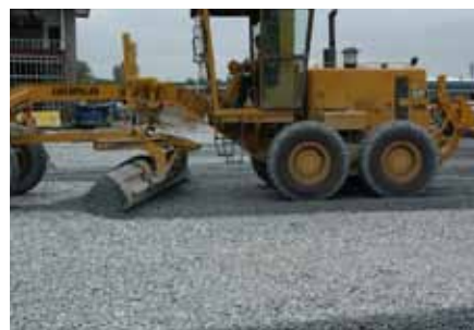
6. Upper sub-base is graded to elevation and compacted.
